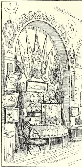
PART OF THE MAURITIUS COURT.
